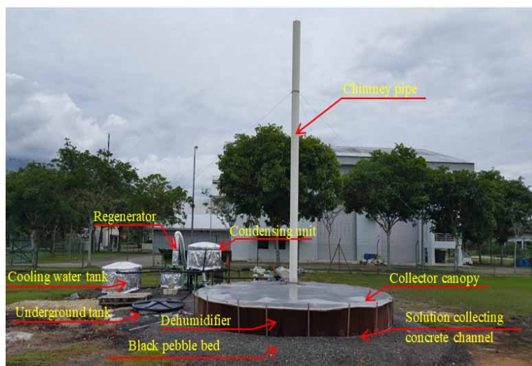
Fig. 5. Photograph of the pilot hybrid plant.
